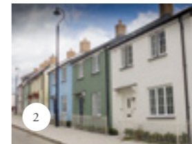
2 NEWQUAY The Duchy’s major development project in Cornwall, Nansledan.
