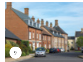
9 POUNDBURY An urban extension to Dorchester, Poundbury is built on principles of architecture and urban planning advocated by The Prince of Wales.
